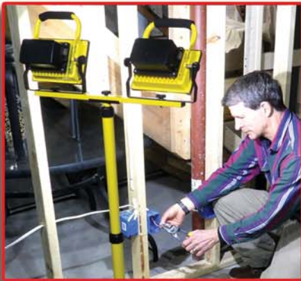
Job sites without electricity
